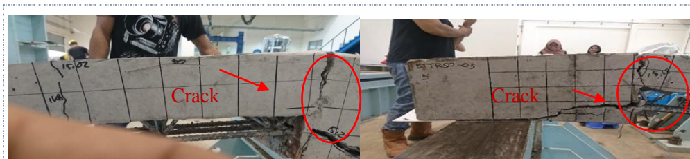
Figure 2. The crack at support.
